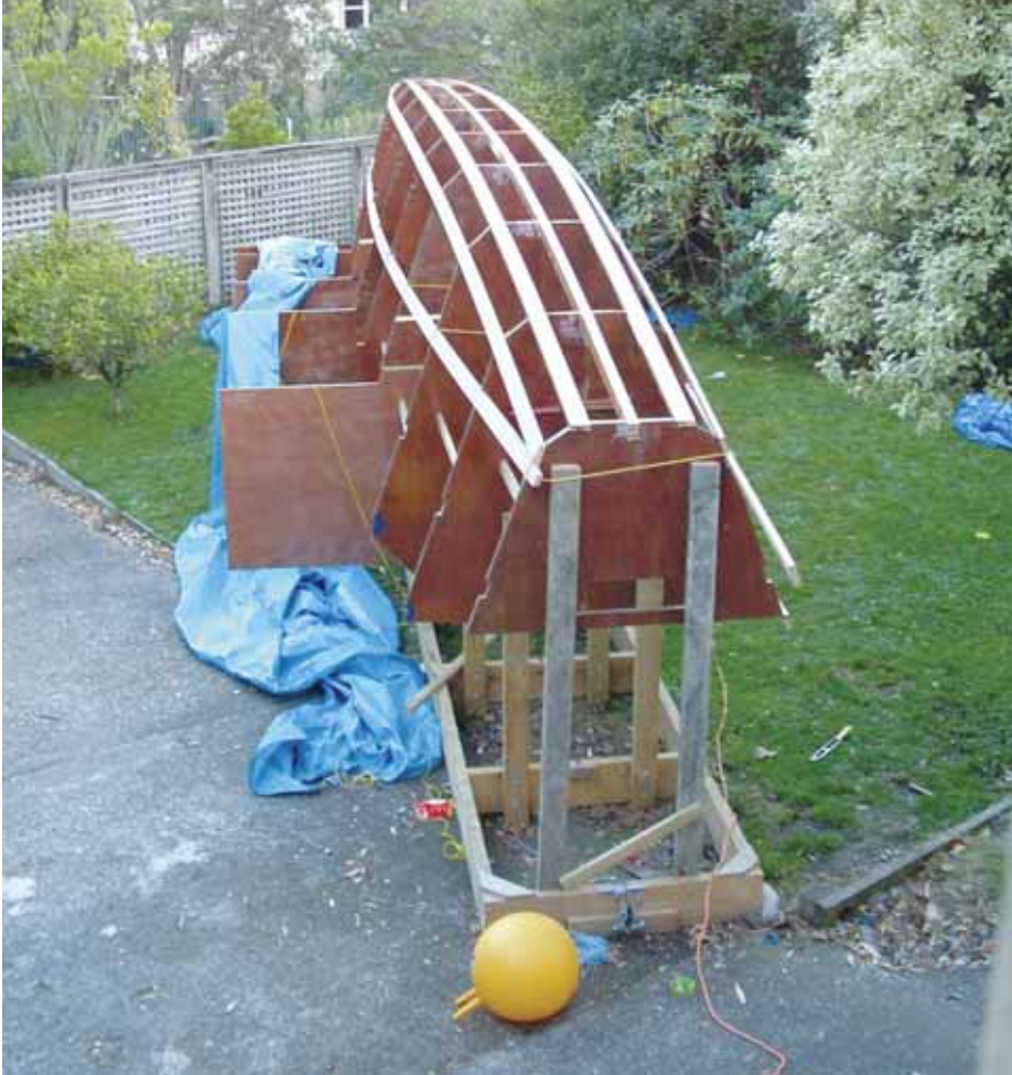
The start of many scarph joints. (left) A framework full of potential. (below)
