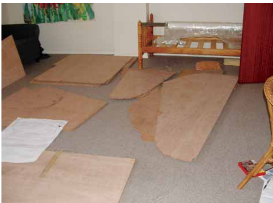
Marking and cutting out bulkheads.
