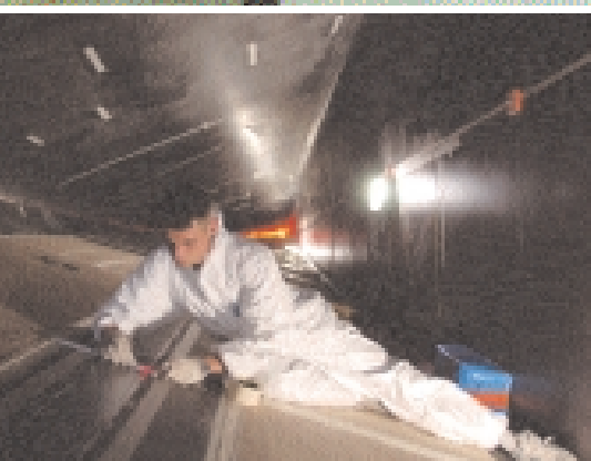
Early stages of the construction. From top to bottom: A half of the central hull plug lays on its side; Crossbeams pre-shapes, show their smooth curves, while a glance is enough to notice how sharp the bows of the floats will be (not unlike the Groupama 2 60 footer, actually); working in central hull.
