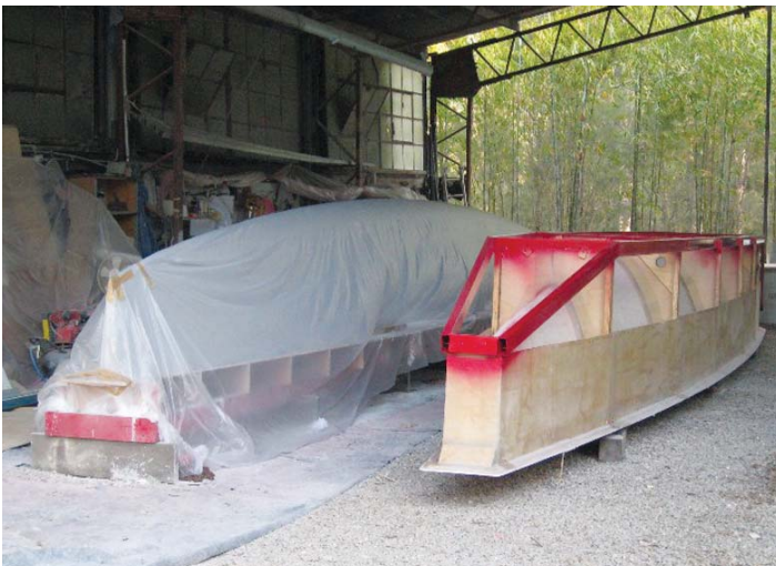
Hull shoe plug (left) and mould (right).
